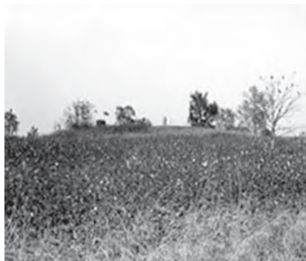
Figure 4-1. Mound A from southwest, 1941.
