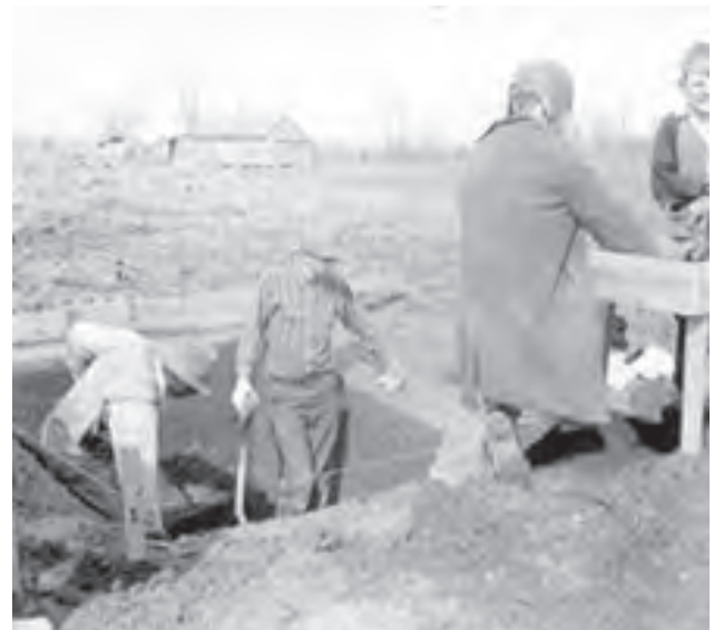
Figure 4-9. Excavation in progress, Section A-VII.
